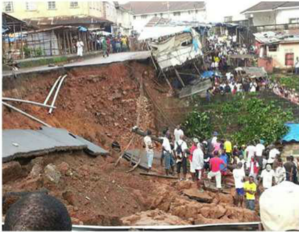
Recent landslide at King Jimmy resulting from bridge failure
